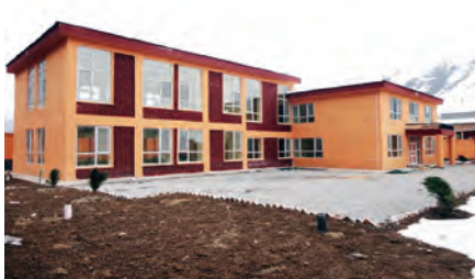
Provincial council administrative building completed under GPI in Panjshir Province, August 2017. (MCN Photo)
