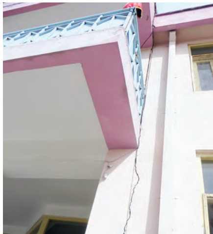
Vertical crack in the facade of Bakhtnoor Bakhtiar School, Khowst Province. (SIGAR photo)
