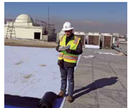
A SIGAR inspector checks work at the new Afghan Ministry of Defense headquarters. (SIGAR photo)
