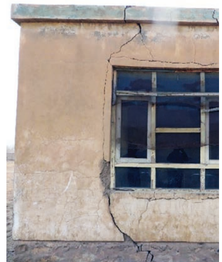
Large cracks in the wall of a school in Baghlan Province. (SIGAR photo)
