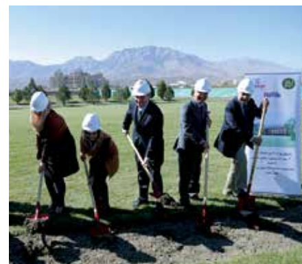
Members of the American University of Afghanistan board of trustees, U.S. officials, and others participated in a groundbreaking ceremony for a 3,000 square-meter women's dormitory in October 2015. The dormitory was opened in January 2018. (USAID photo)
