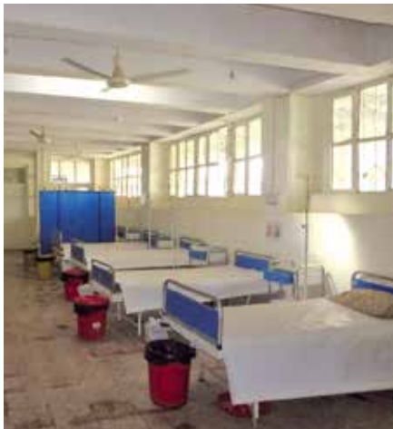
A structurally sound and clean infirmary in Kandahar Province. (SIGAR photo)
