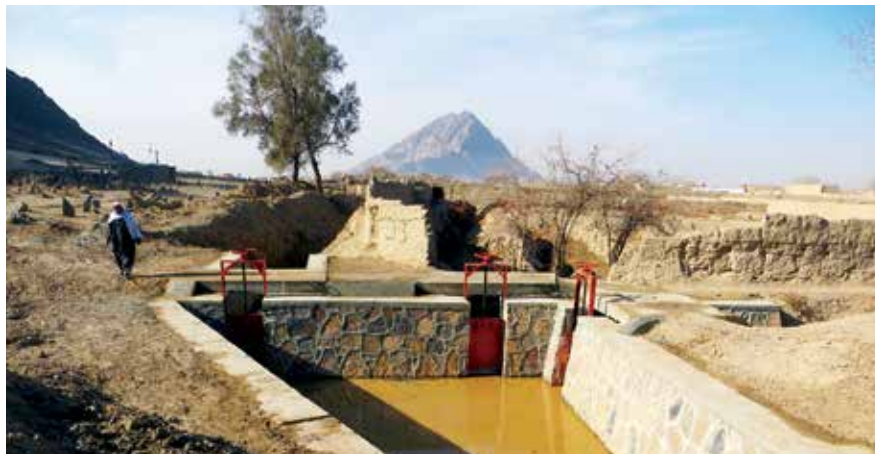
Salawat irrigation canal in Kandahar Province. (USAID photo)
